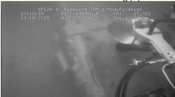
Using underwater positioning to fix the cutting point
