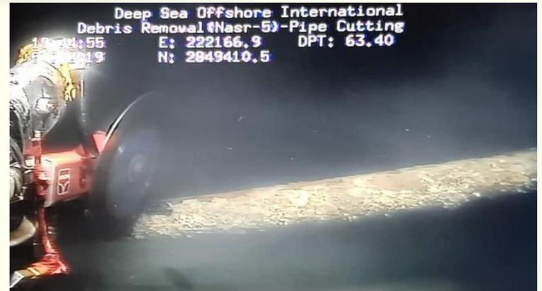
Start cutting pipe using hydraulic cutter
