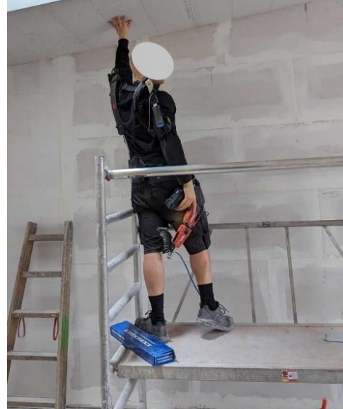
Figure 2. Example of position requiring a complex arm position for the exoskeleton.
